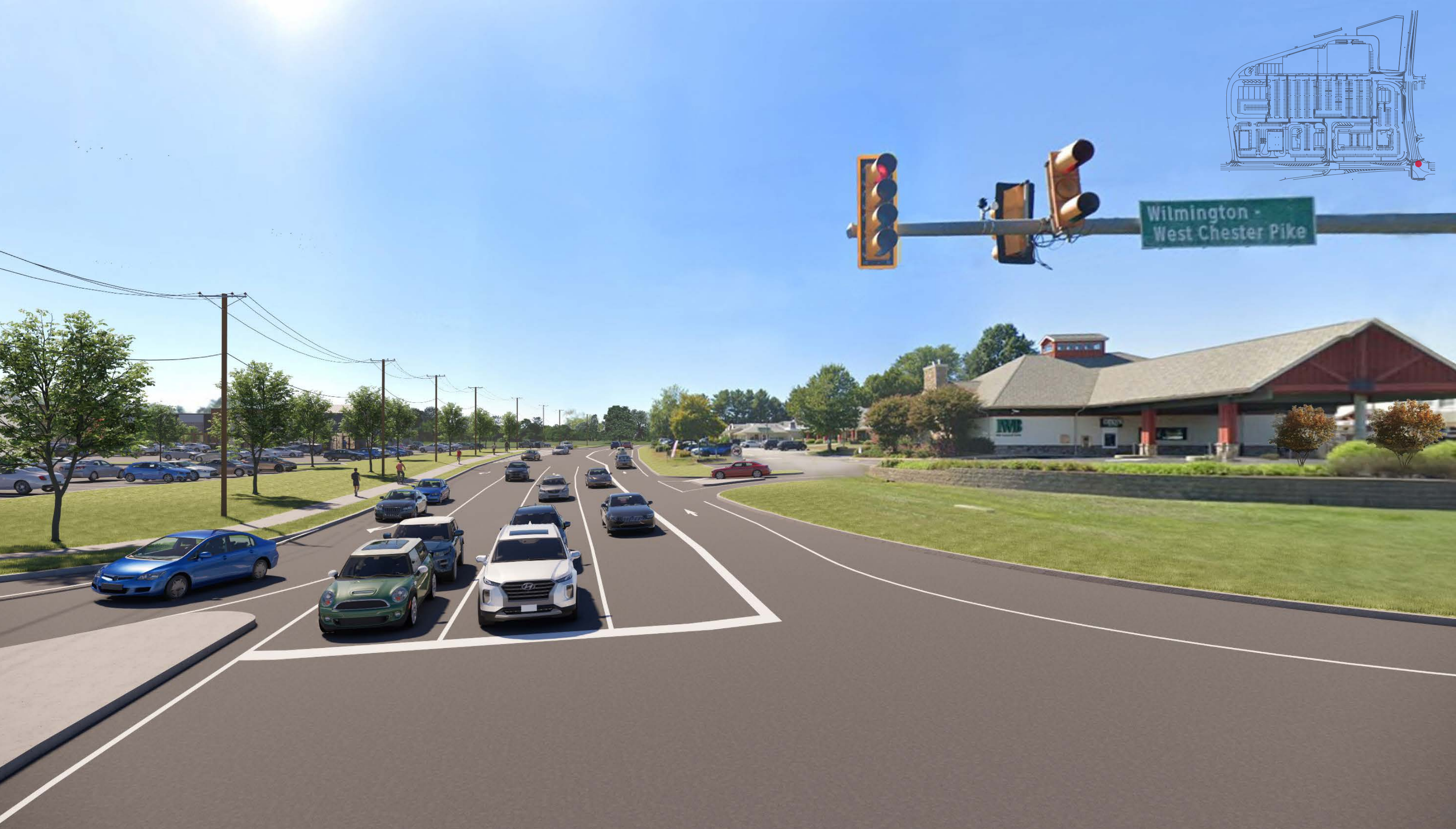
Ridge Rd Improvements - Westchester Pike View
